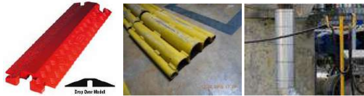
Figure 8. 1 Example of Metal Cover & Hanger for Electric Cable
