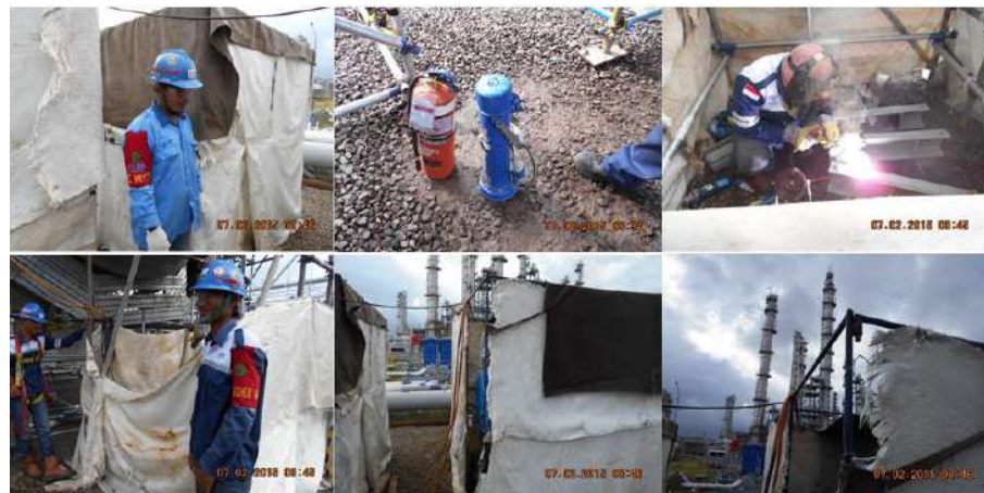
Figure 12. 1 Hot Work Class I Requirement (Fire Watchman, FE, PPE, Shelter) Example
